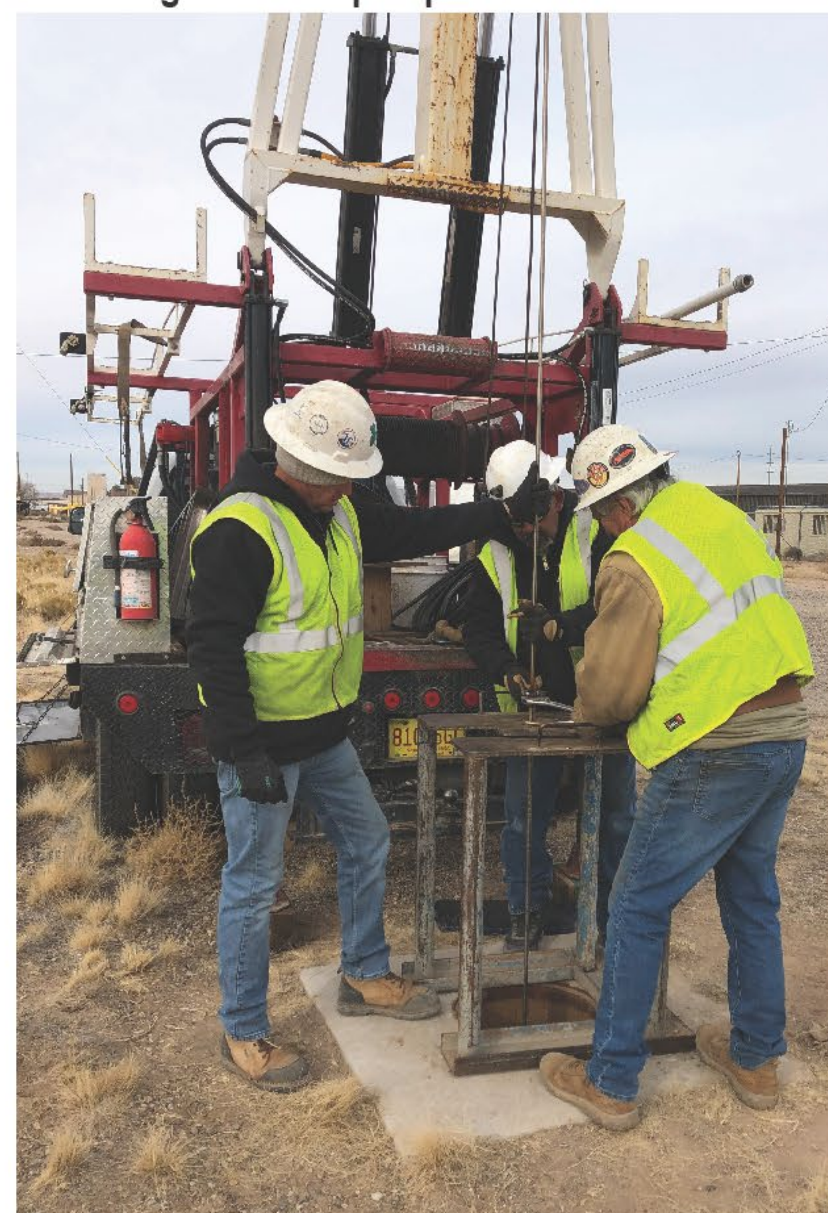
Removing the failed pump in KAFB-106024
