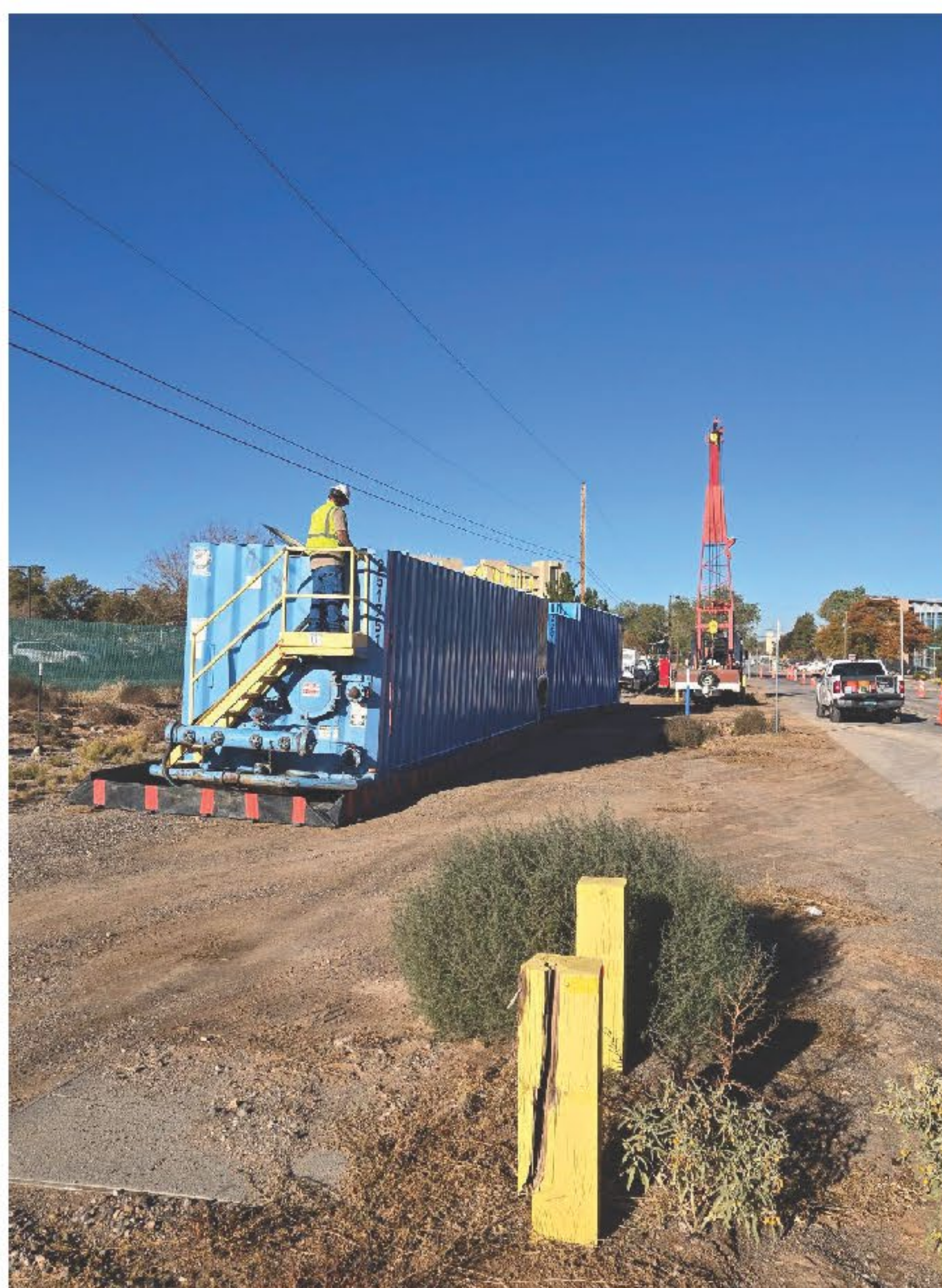
Extraction well KAFB-106239 rehabilitation
