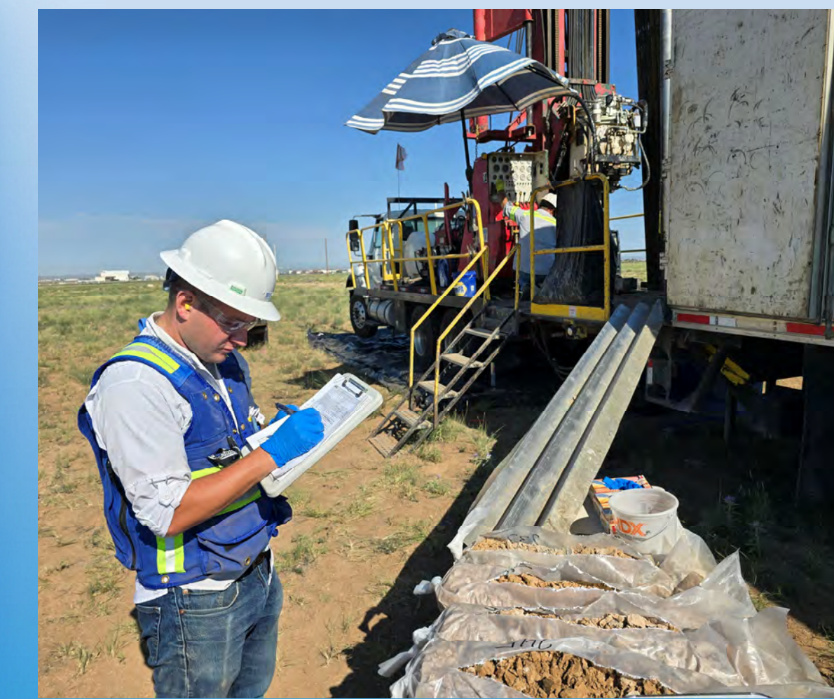
Installation of KAFB-WYO-5
