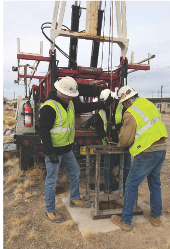
Removing the failed pump in KAFB-106024
