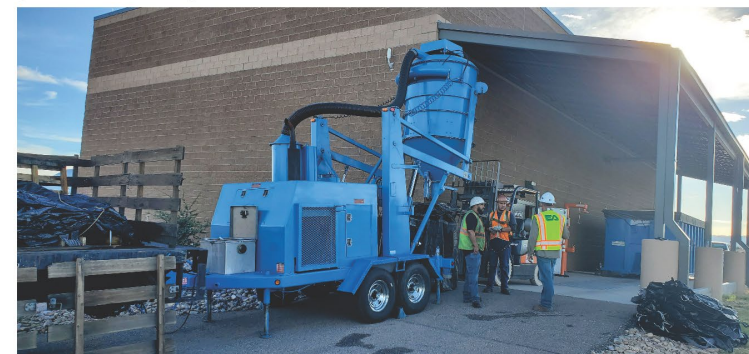
Preparation for carbon change out at the groundwater treatment system
