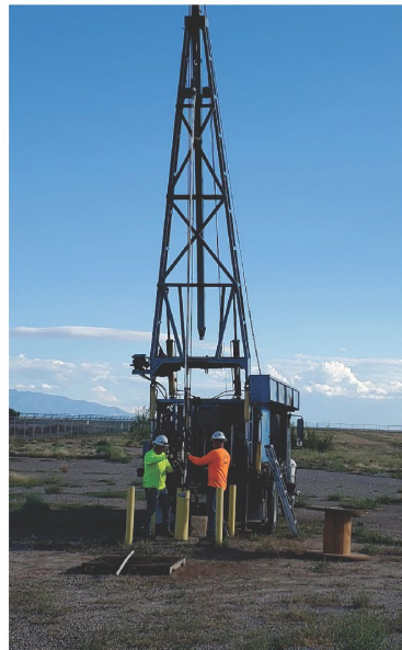
Performing pump stinger installation
