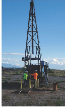
Performing pump stinger installation
