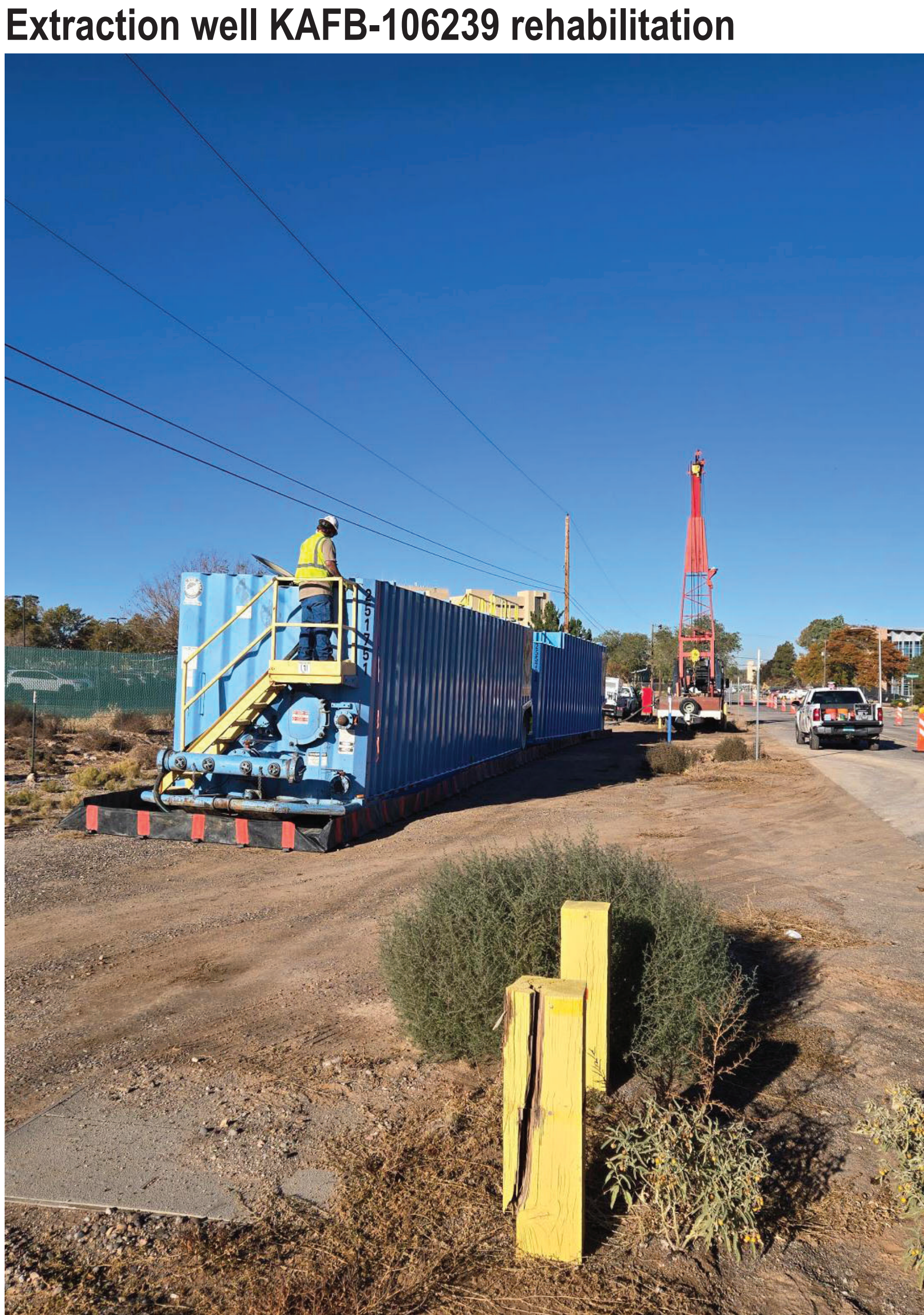
Extraction well KAFB-106239 rehabilitation
