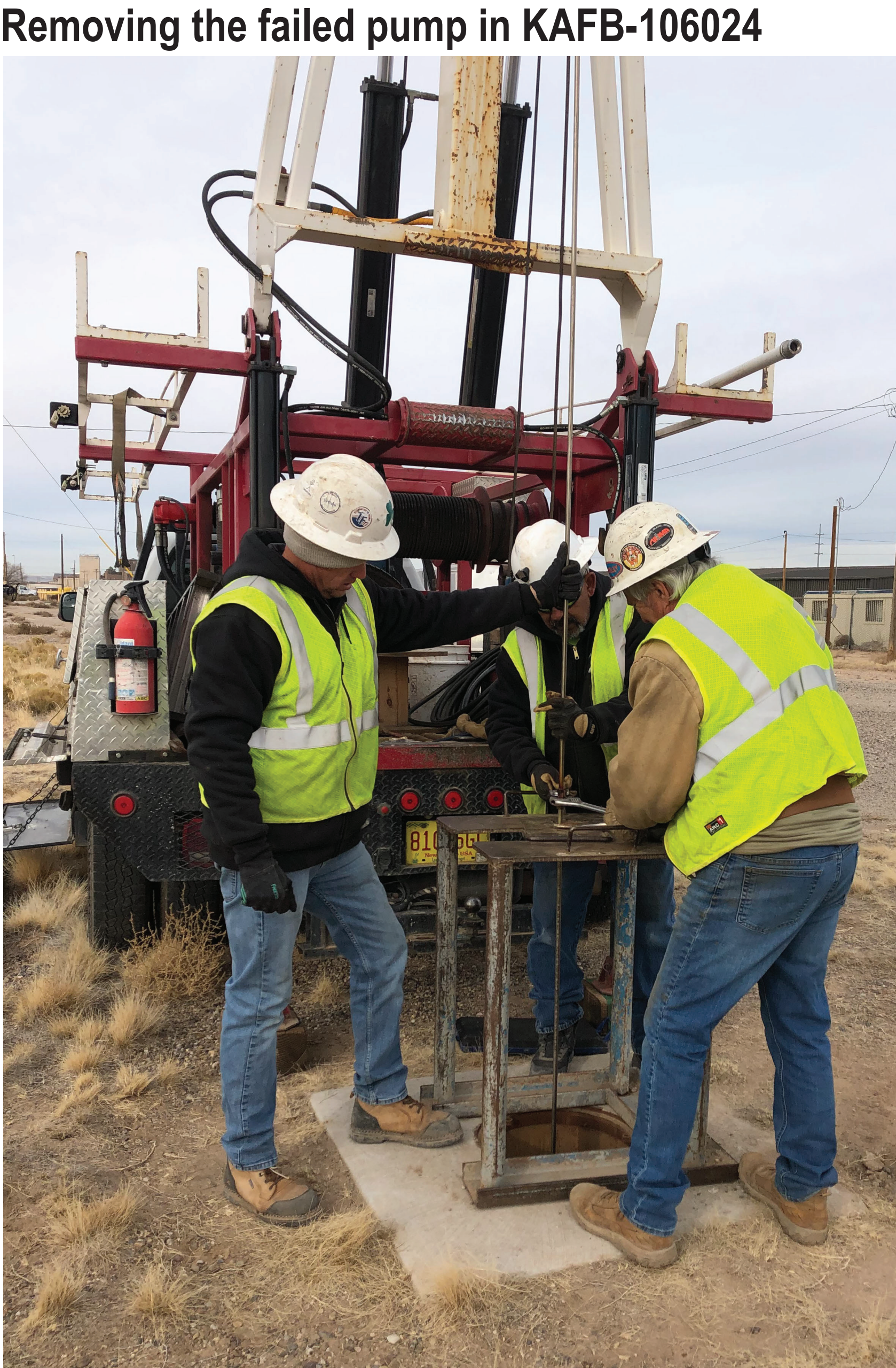
Removing the failed pump in KAFB-106024
