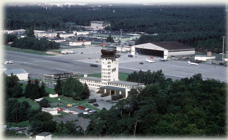
The Air Control Tower at Ramstein AB, ca. 1980s. (USAF Photo)
